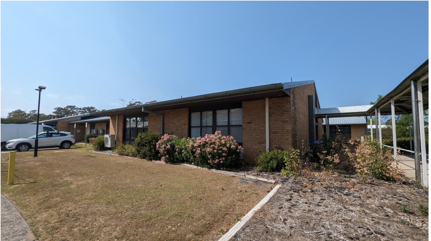
Figure 6 – Block C - Wyong Hospital looking along the northern elevation
