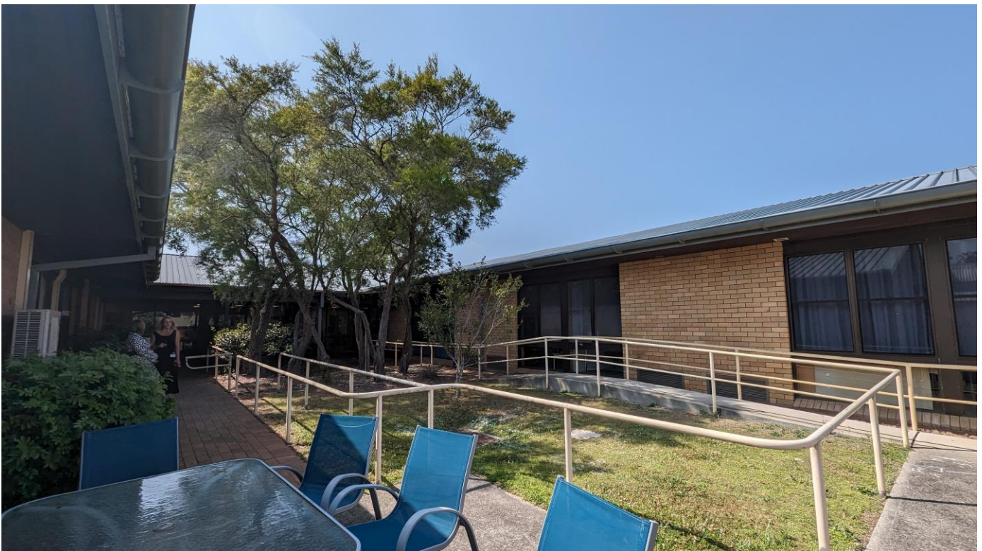
Figure 3 – Block C - Wyong Hospital looking into the central courtyard area
