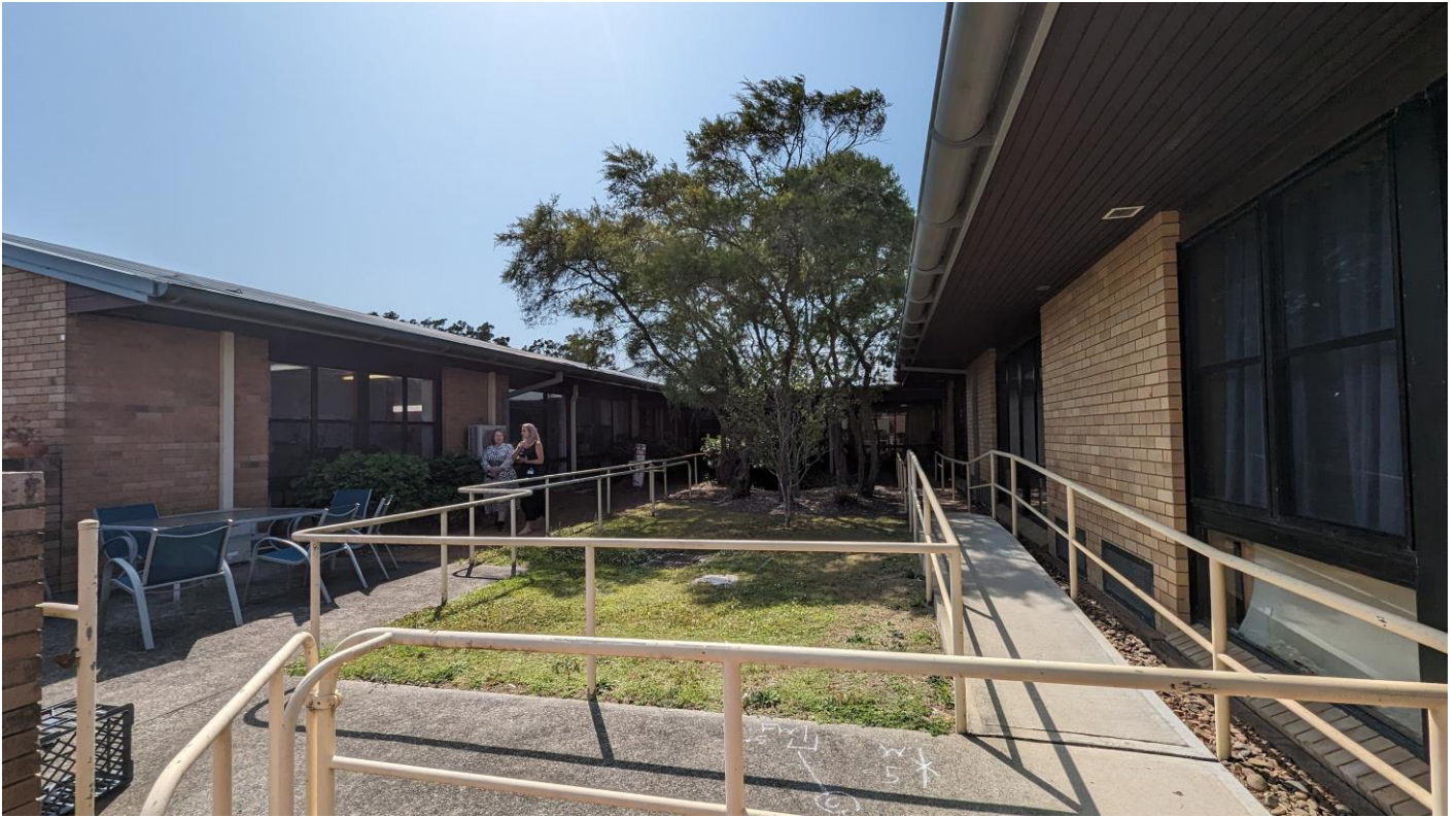
Figure 4 – Block C - Wyong Hospital looking into the central courtyard area
