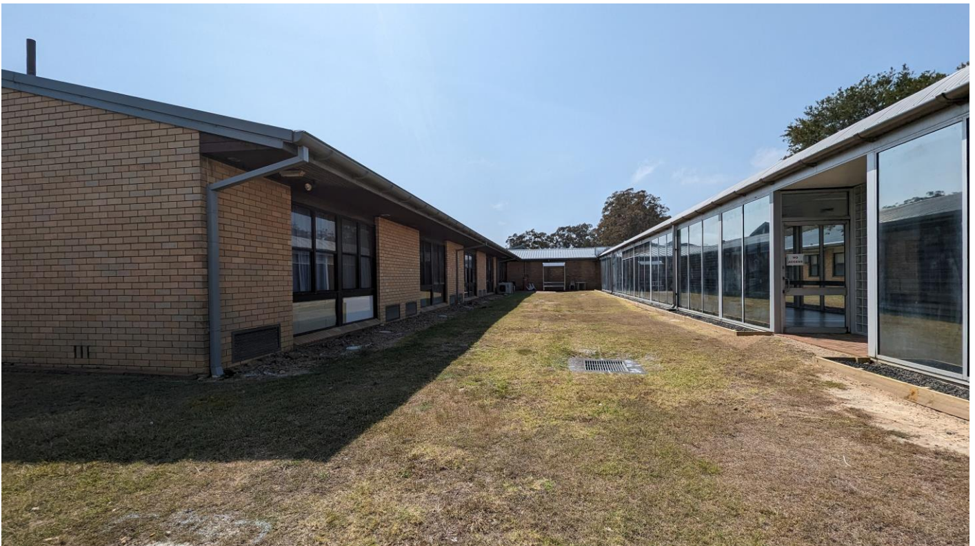
Figure 5 – Block C - Wyong Hospital looking along the southern elevation
